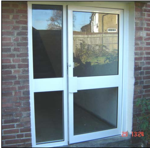
New security door at Shaftesbury Circle
